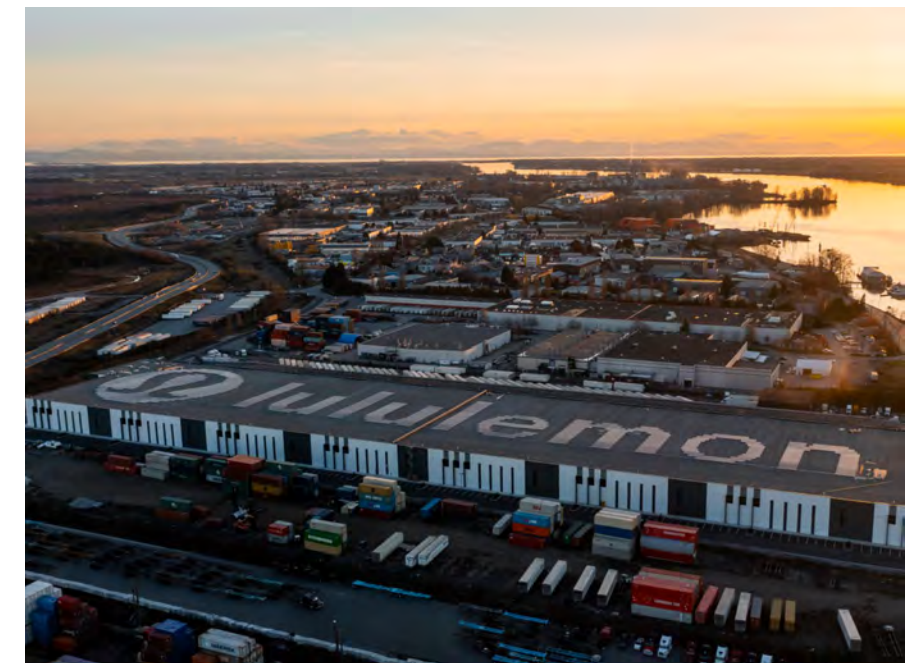
Solar panels on our Delta distribution centre.
